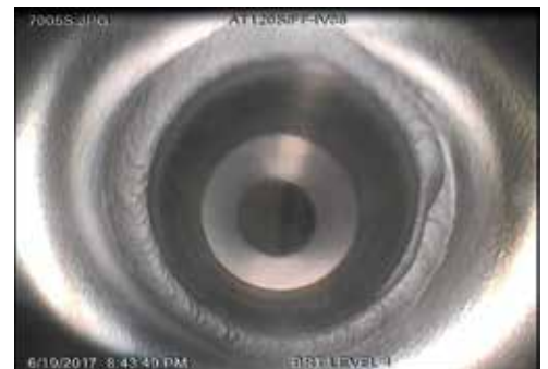
Borescope inspection view
